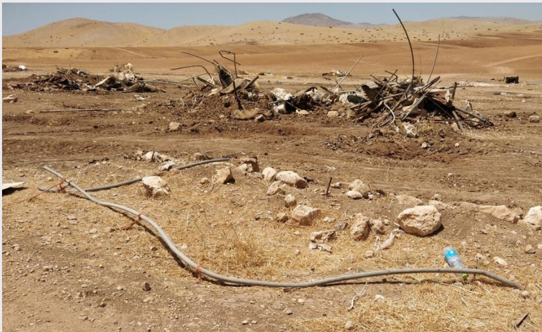
Homsa, after demolition, July 21, 2021. Photo: Daphne Banai
